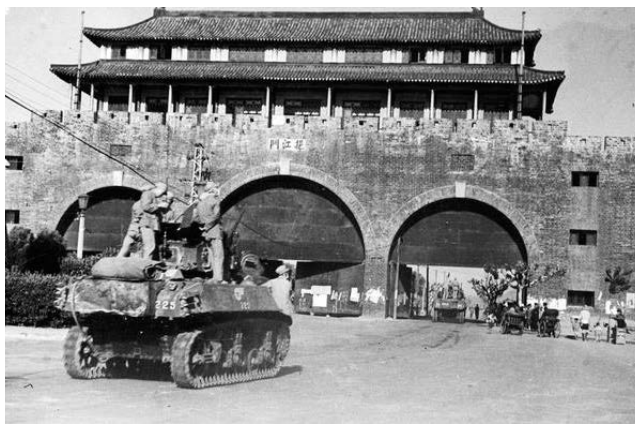
Fig. 2 Photo of the Yijiang Gate 圖2 掘江門照片
